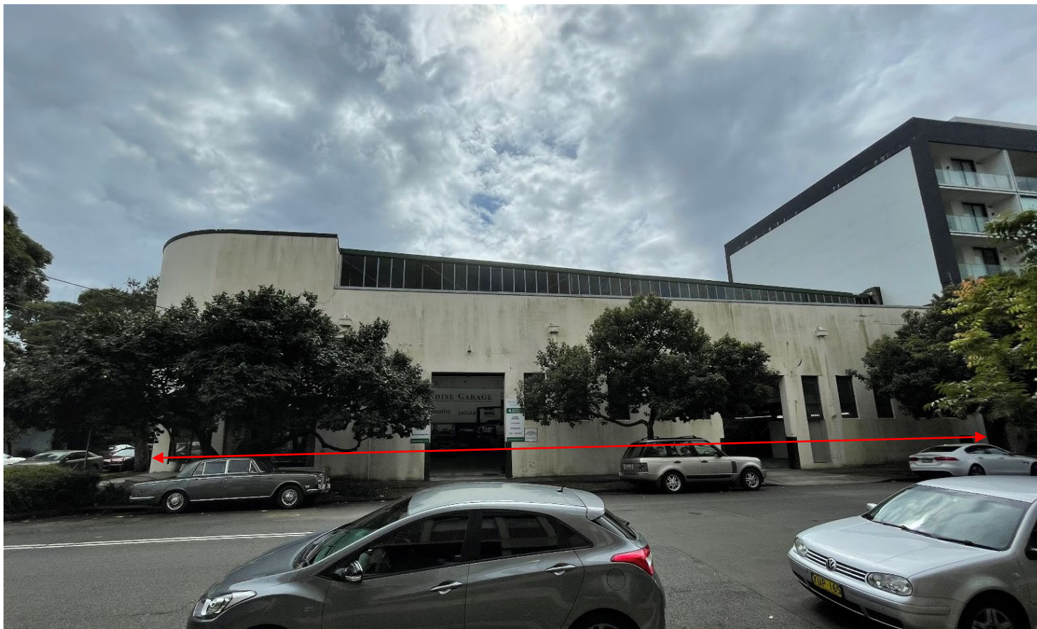
Cressy Street frontage
