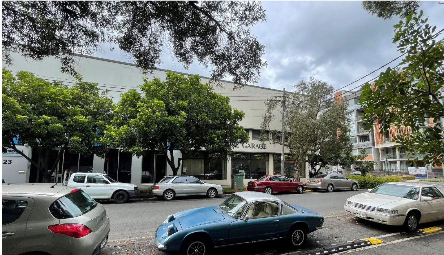
Dunning Avenue frontage
